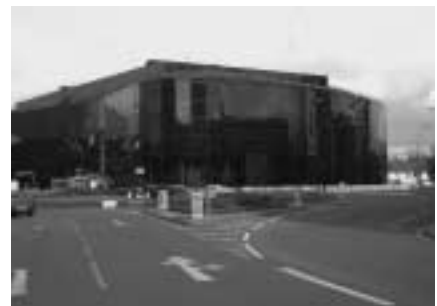
The Willis Coroon Building
